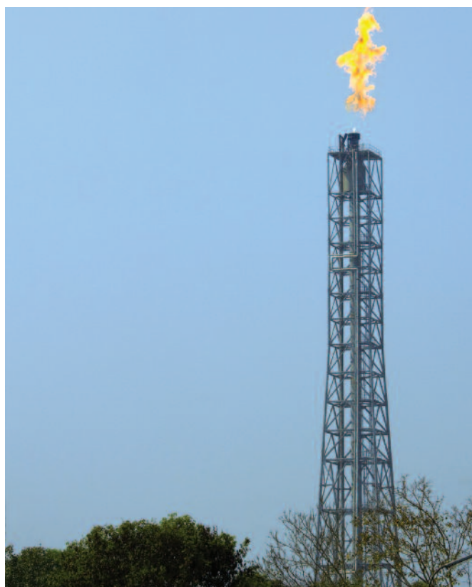
A flare stack burning off excess gas at the Mathura Refinery near Agra, India. © Sundeep/Shutterstock
