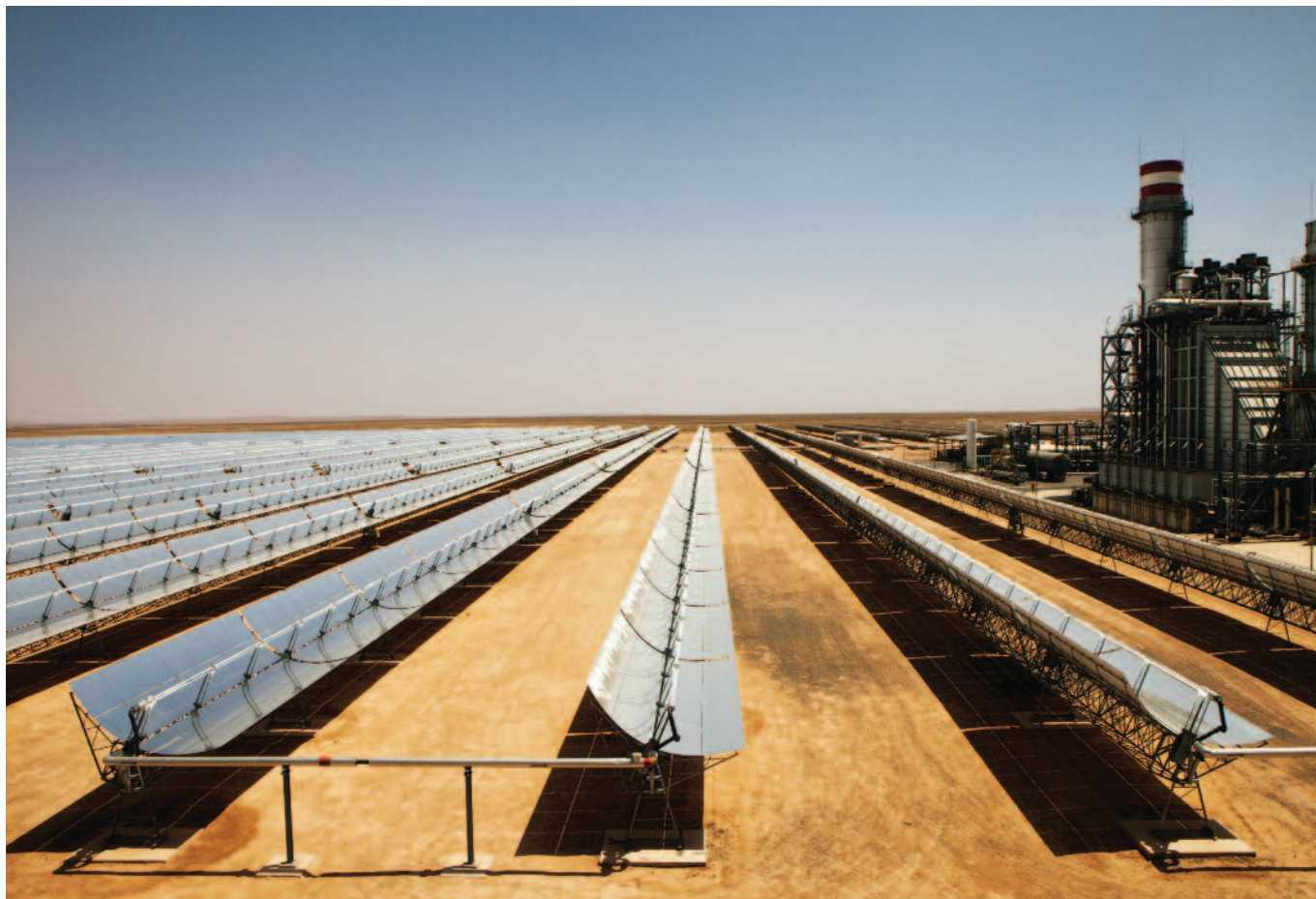
Alternatives to fracking. The Ain Beni Mathar Solar Plant in Morocco. The solar plant is the first hybrid combined solar cycle plant worldwide. It has a 470 MW capacity and avoids 33,000 tonnes CO 2 emissions per year.
