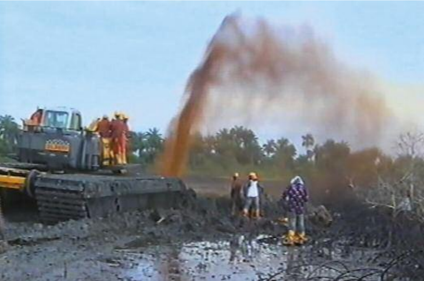
Shell workers arriving to clamp the broken pipeline, Bodo, 7 November 2008.
