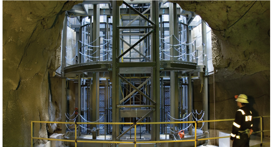
Sinking of the #10 shaft is underway
