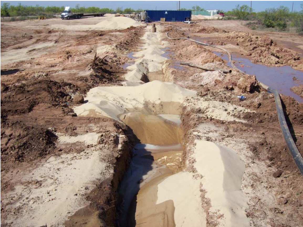
Figure 1 Installation of the Receptor Trench
