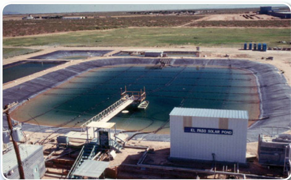
Figure 7. Photograph of a salinity gradient solar pond (Karl Longley, California Regional Water Quality Control Board).
