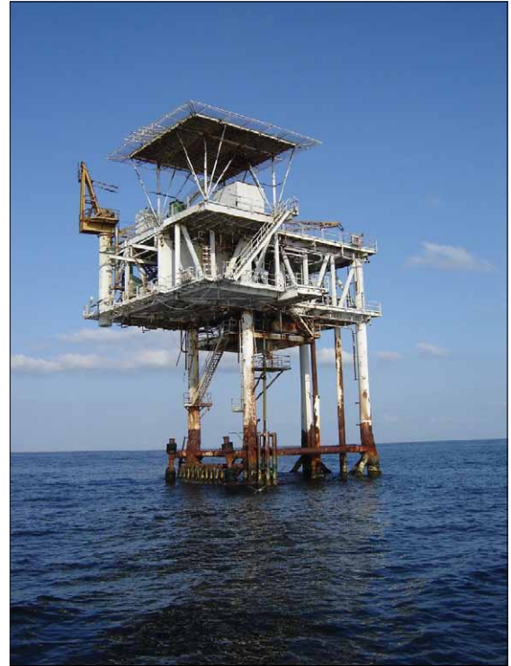
Offshore Rig in the Gulf of Mexico
