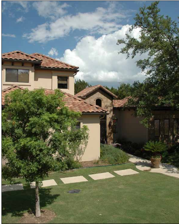
Residence with underground propane tank
