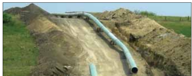
Transmission pipeline construction project near Fort Worth
