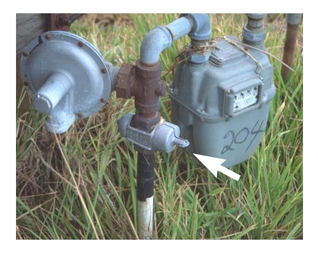
Below is an example of a service that has been shut off (note position of meter valve) but not locked to prevent opening. This <u>DOES NOT</u> meet the pipeline safety regulations.
