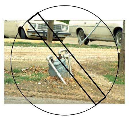
Service regulators installed inside a building must be placed as close as practical to the point of service entering the building. The operator must vent the regulator to the outside.
