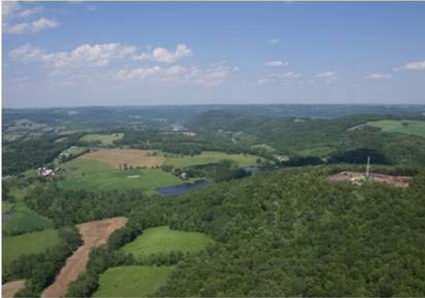
Photo 5.5 Chesapeake Energy Marcellus well drilling, Bradford County, PA Source: Chesapeake Energy
