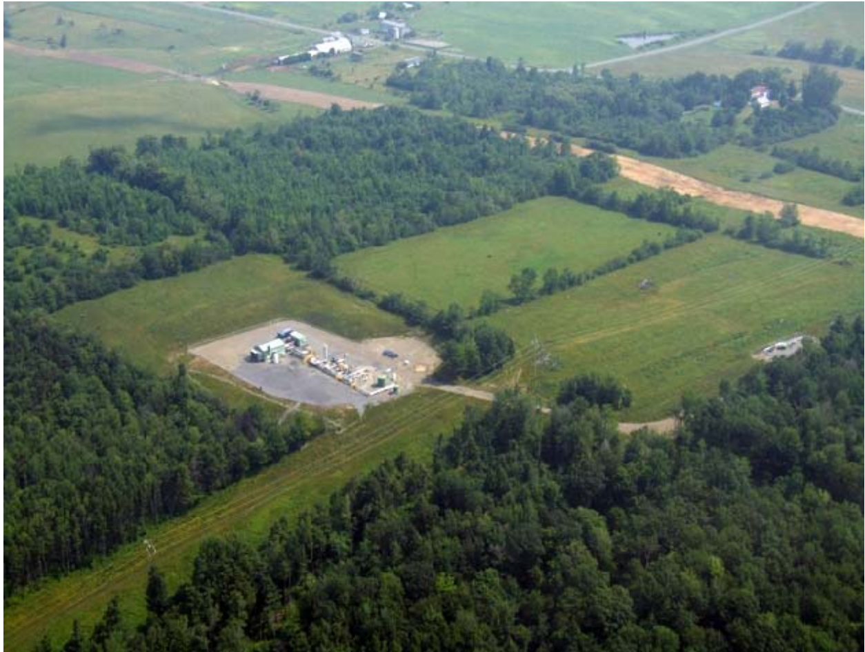
Photo 5.28 - Pipeline Compressor in New York. Source: Fortuna Energy
