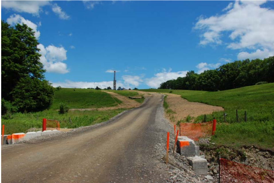
Photo 5.1 Access road and erosion/sedimentation controls, Salo 1, Barton, Tioga County NY. Photo taken during drilling phase. This access road is approximately 1,400 feet long. Road width averages 22 feet wide, 28 feet wide at creek crossing (foreground). Width including drainage ditches is approximately 27 feet. Source: NYS DEC 2007.
