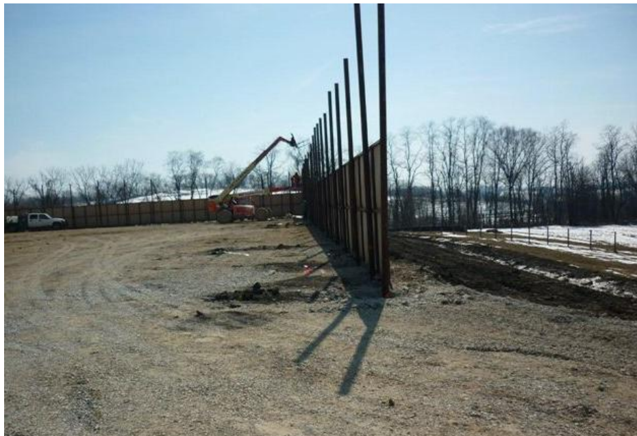
Photo 7.4 - Sound Barrier Installation (New August 2011)
