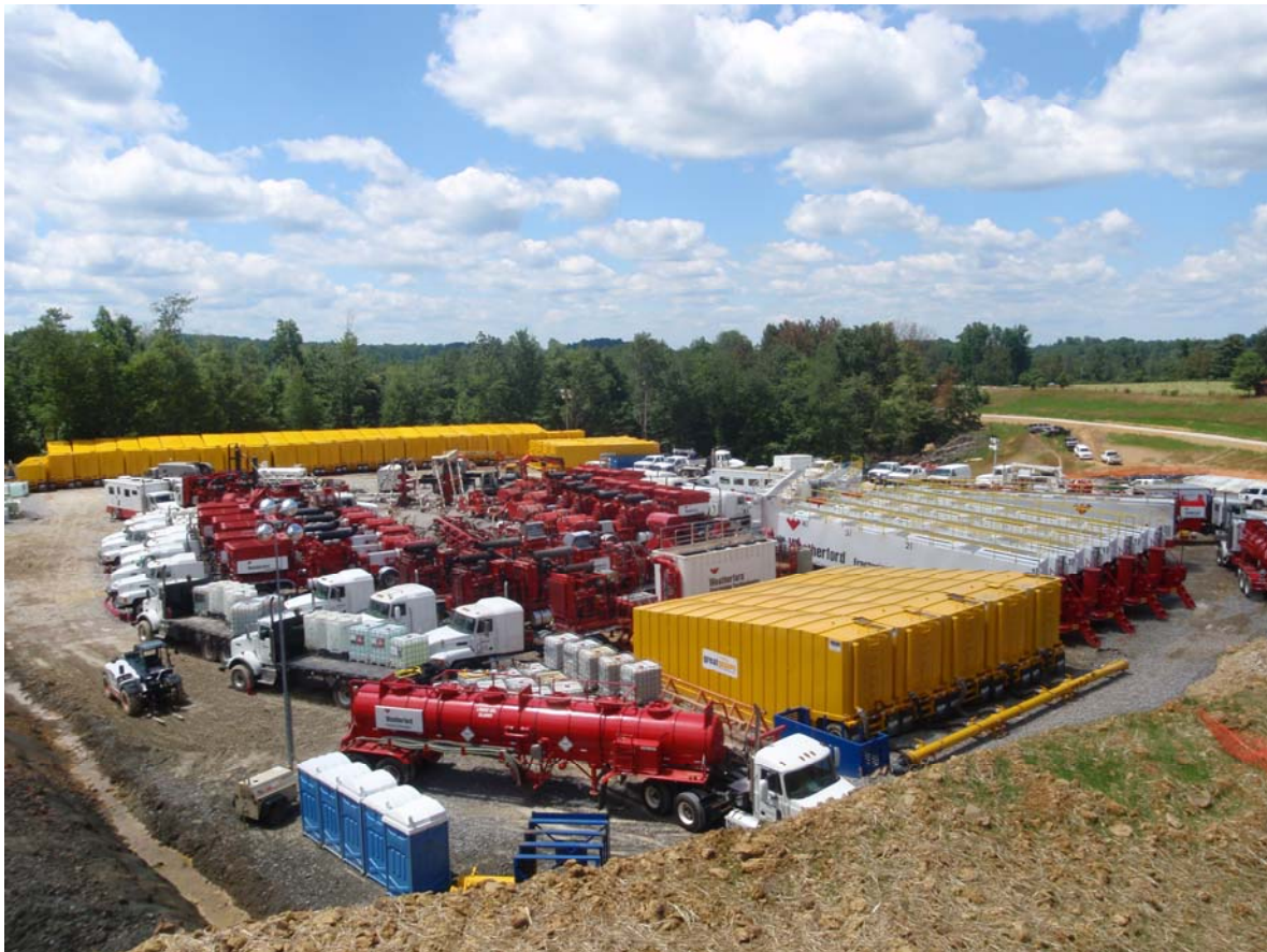
Photo 5.6 Hydraulic fracturing operation, horizontal Marcellus well, Upshur County, WV Source: Chesapeake Energy, 2008
