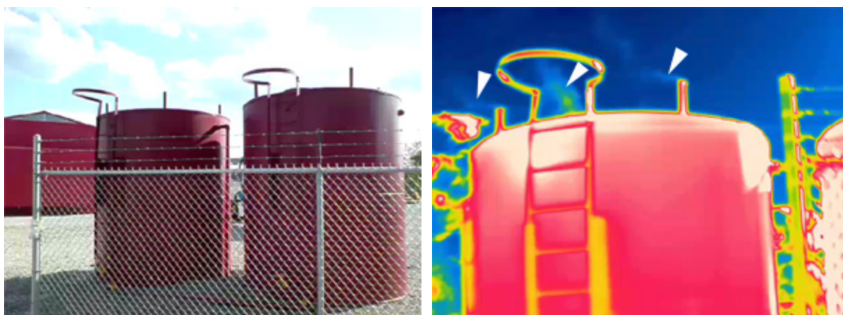
Figure 9: FLIR images of the heavy condensate tanks at the Energy Corp. Compressor Station. Gas emissions are referenced by the white arrows.
