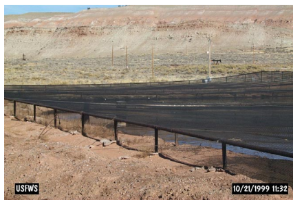
Proper netting of oil pits can exclude wildlife and prevent mortality. Photo by Pedro Ramirez, Jr./USFWS
