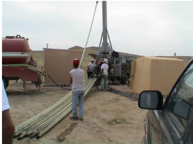
CBM Drilling Operations - Wyoming
