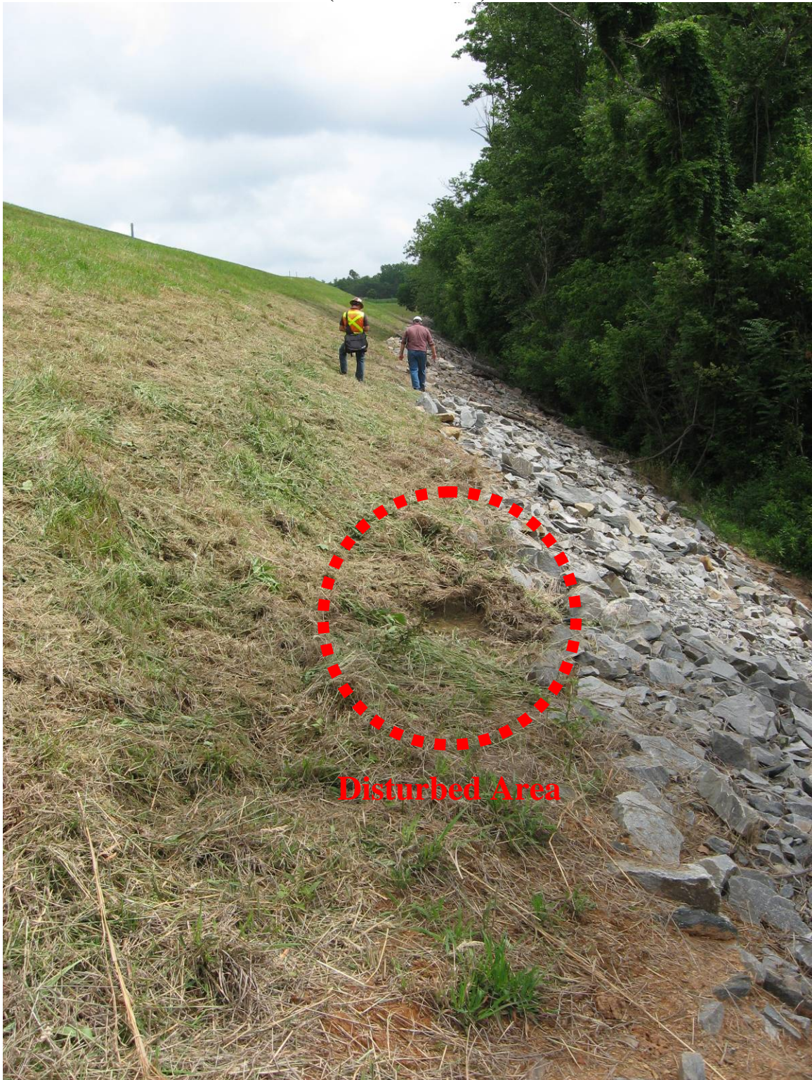
PHOTO 7: SOUTHERN EMBANKMENT SECTION OF PRIMARY POND (LOOKING NE)
