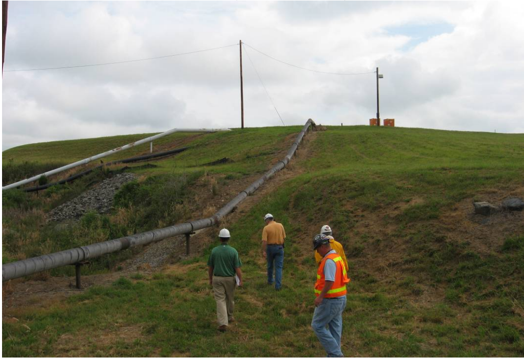
PHOTO 3: SOUTHWEST CORNER OF PRIMARY POND WITH SLUICE LINES (LOOKING NE)
