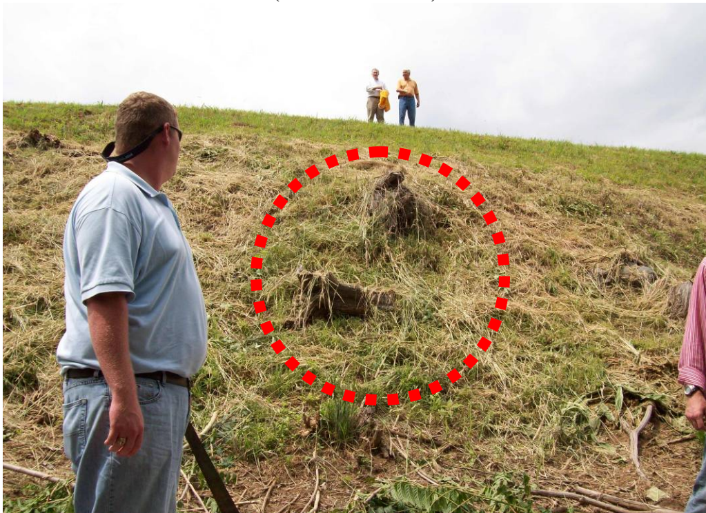
PHOTO 6: STUMPS IN PRIMARY POND SOUTHERN EMBANKMENT SLOPE (LOOKING NW)
