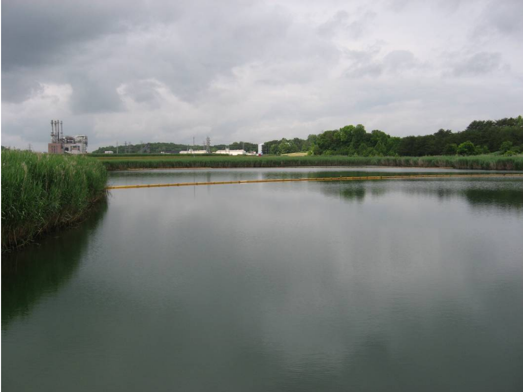
PHOTO 13: VIEW ACROSS PRIMARY POND FROM PRIMARY DISCHARGE TOWER (LOOKING SW)
