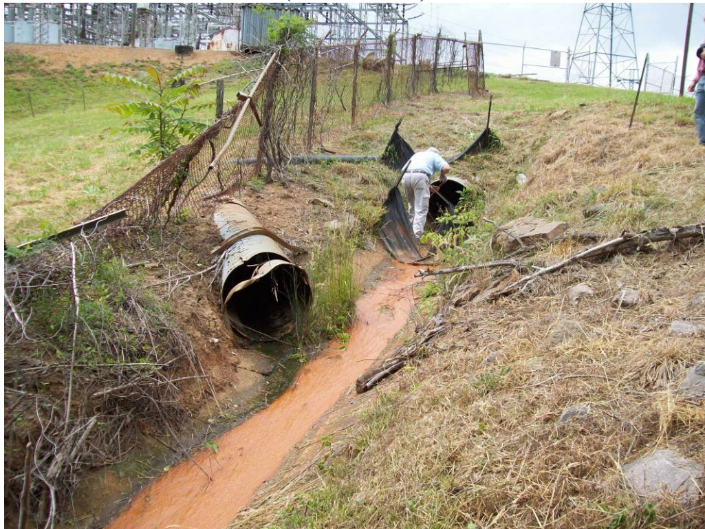
PHOTO 2: SURFACE DRAINAGE OUTFALL BETWEEN PLANT AND POND (LOOKING N)
