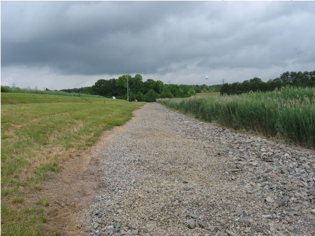
PHOTO 12: INTERMEDIATE DIKE CREST (LOOKING NW)
