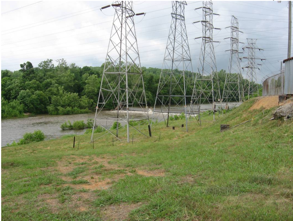
PHOTO 1: LOW HEAD DAM IN DAN RIVER (LOOKING SW)
