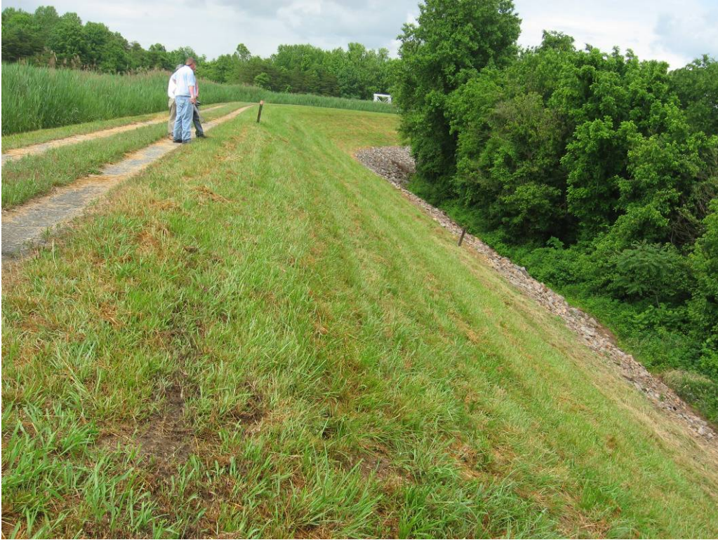
PHOTO 15: SOUTHERN EMBANKMENT OF SECONDARY POND (LOOKING NE)
