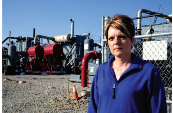
Pam at the compressor station near her home.
