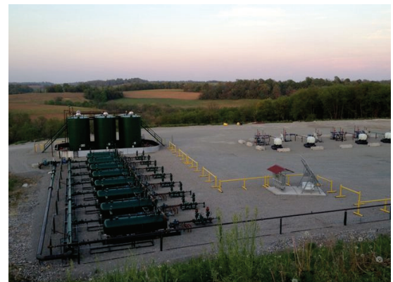
Separators split off heavy hydrocarbons from gas, and often vent methane and volatile organic compounds into the air.
