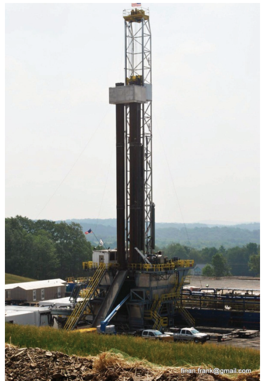
Drilling rig onsite.
