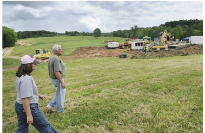
Linda and David watch pipeline construction across their hayfields.
