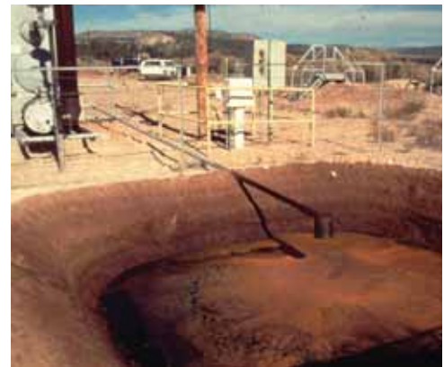
FIGURE I-9. WASTE PIT Waste pits for fluids and sediments associated with gas processing. These can contain water, sand, hydrocarbons, glycol and other chemicals.
