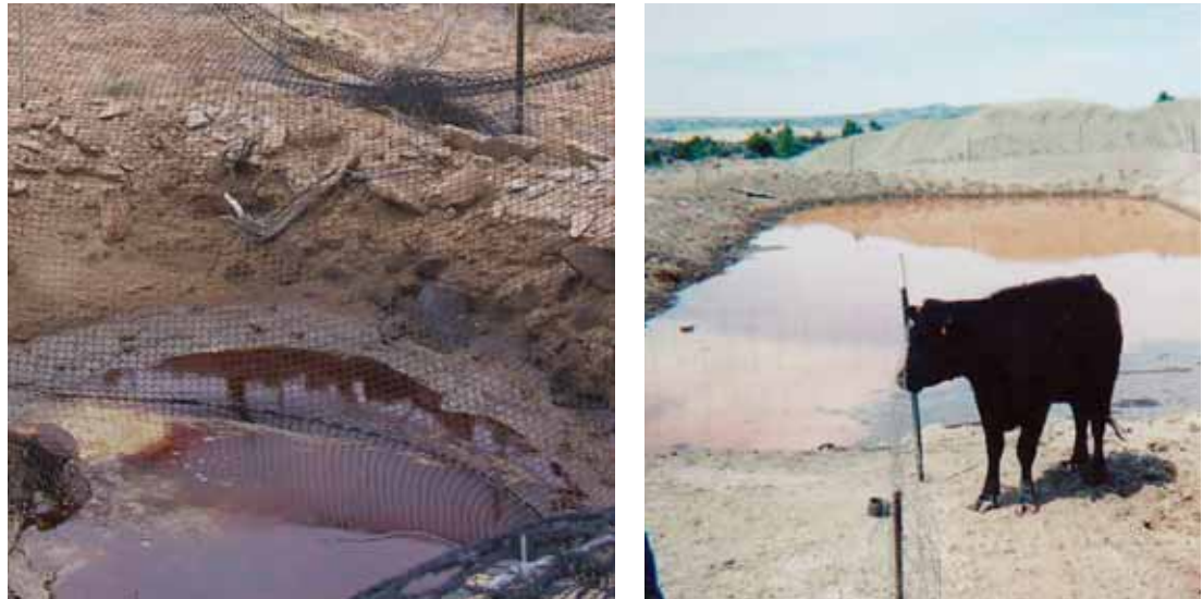
FIGURE I-27. IMPROPER NETTING AND FENCING Can result in death of wildlife and livestock.
