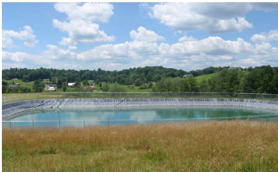
Photo 5.22 Construction of freshwater impoundment in Upshur Co. WV. Source: Chesapeake Energy
