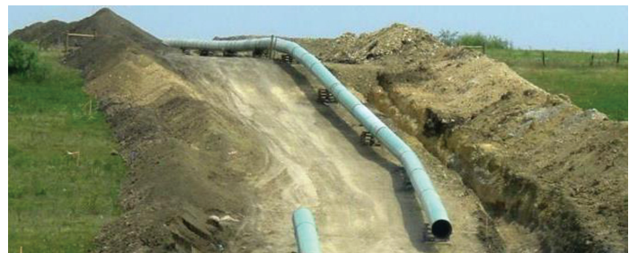
Figure 4-4 Transmission pipeline construction project near Fort Worth
