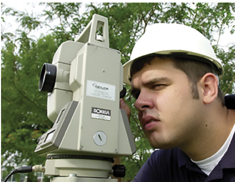
Pipeline civil survey.
