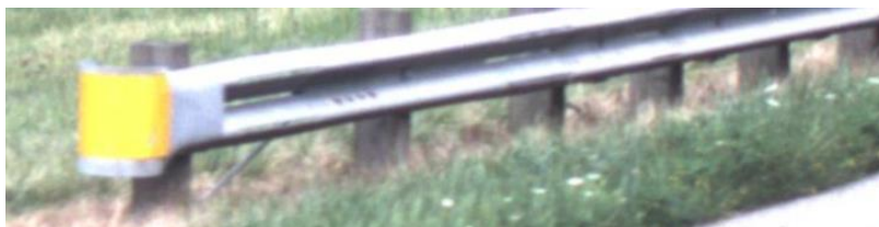
Figure 5. SRT on Interstate 77 in Guernsey County
