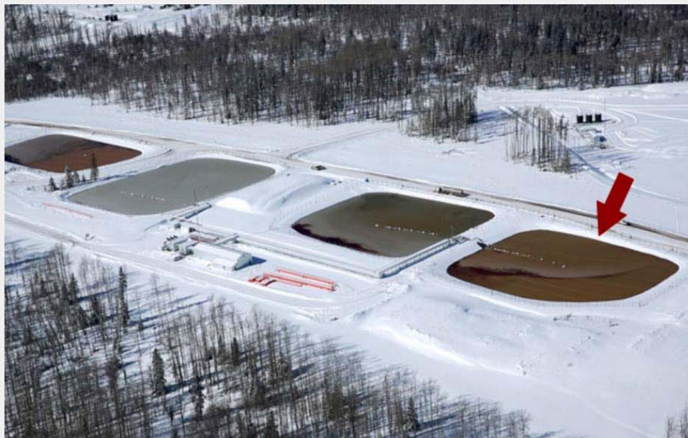
Four frackwater pits in Talisman's Farrell Creek operations in northeast BC – photo taken in March. Pond A, on the far right, suffered a rupture, leaking contaminants into the soil and groundwater (Two Island Films)
