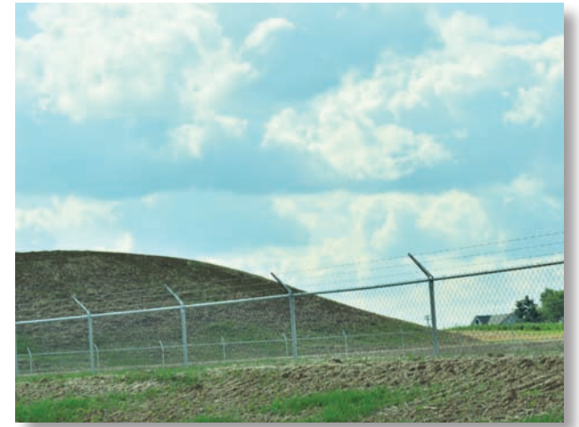
That bulge is where Chesapeake has piled up the Moresheiser’s topsoil to make the pad for their rig.
