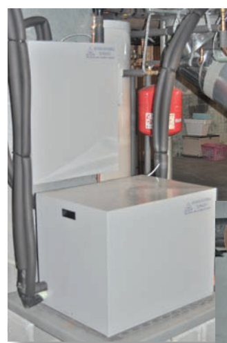
Above: The big box is the heat pump; the box on the wall is the heat exchanger.
