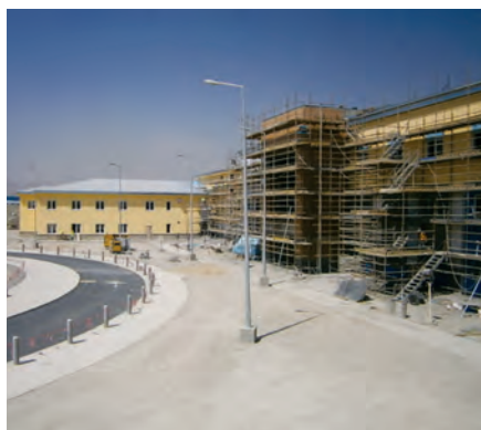
Ministry of Interior headquarters under construction in Kabul, September 2014. (USACE photo)
