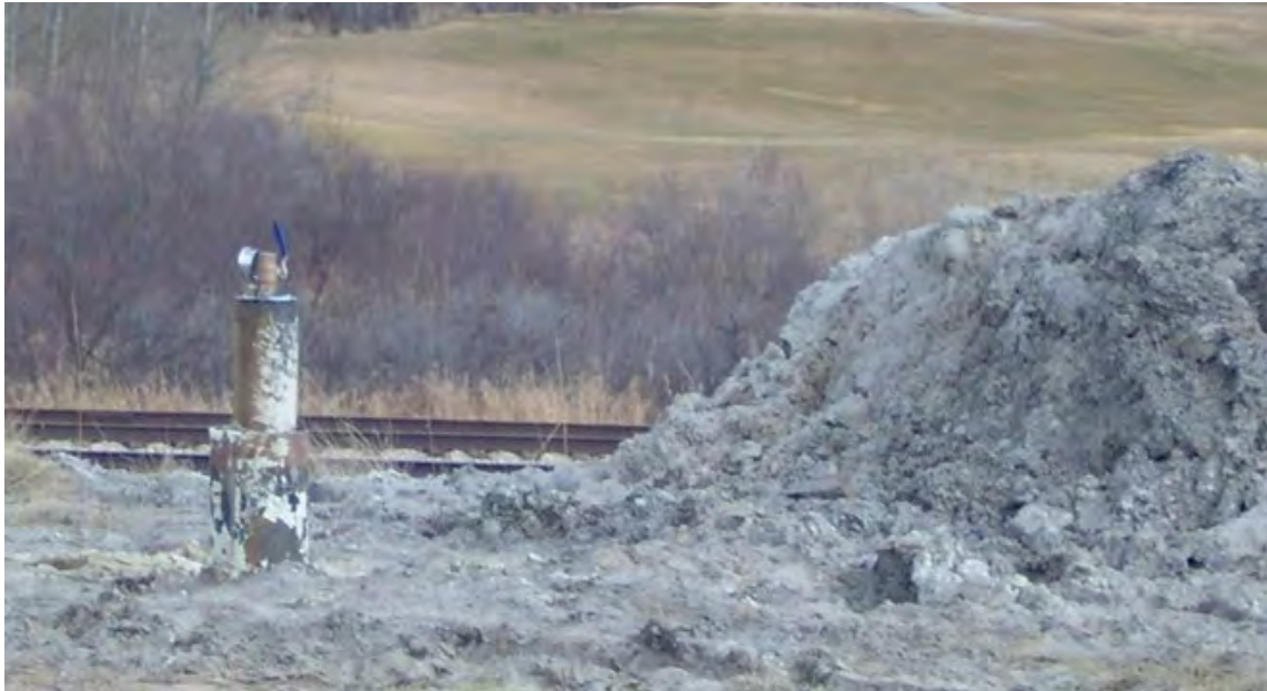
Alberta Environment water monitoring well near a public road in the Hamlet of Rosebud (before compression cap and lock show below), April 2007. The lid was forced open by the venting gas.
