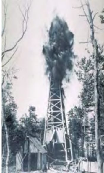
“Fracturing Stoney Creek Field well with nitroglycerin, circa 1940”
