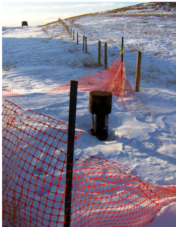
Alberta Environment's water monitoring well in the Hamlet of Rosebud, compression lid and locked to mitigate the danger because this well produces gas instead of water. Alberta's water regulator had to apply to the energy regulator for gas well licensing. A developer plans to build 17 homes at this location.
