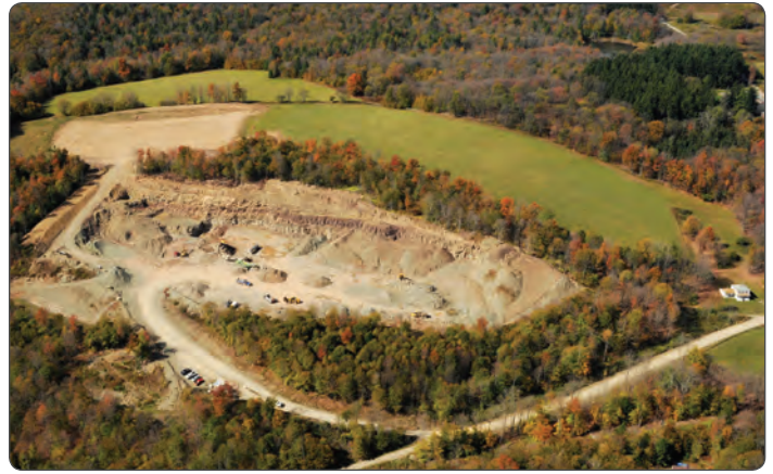
Land is cleared for drilling and fracking in Pennsylvania.
