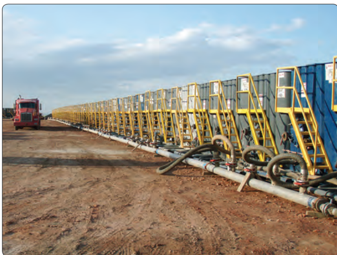
Water tanks lined up in preparation for fracking.
