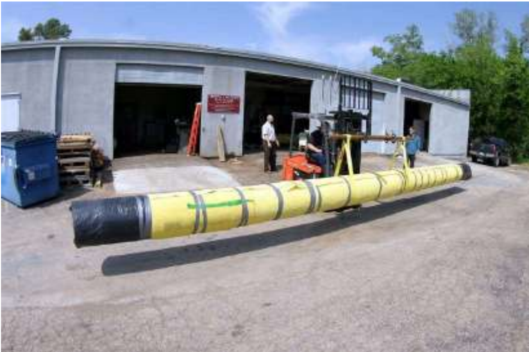
The photographs display two (2) pipe sections during the unloading process. There was no evidence of any transportation related damage to the pipe sections.
