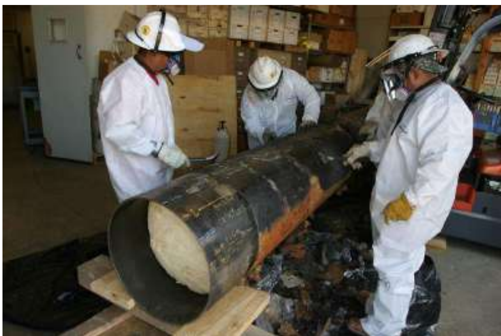
The photographs display the hand removal process of the coating which remained on the pipe after initial removal with hammer.
