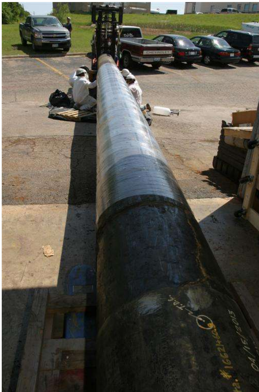
The photograph displays the initial coating removal process.
