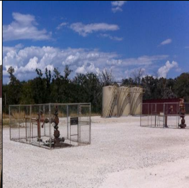
Acme site on 09-02-11
