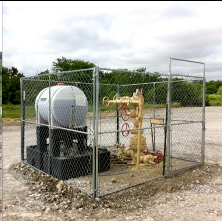
McCutchin 2 well on 05-02-12
