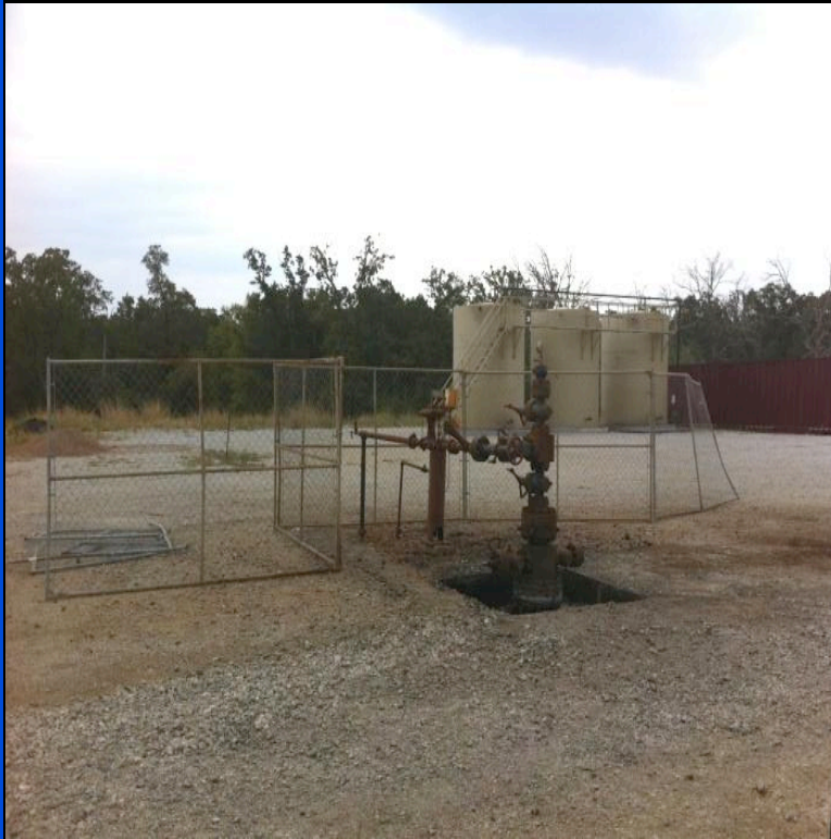
Acme site on 08-29-11
