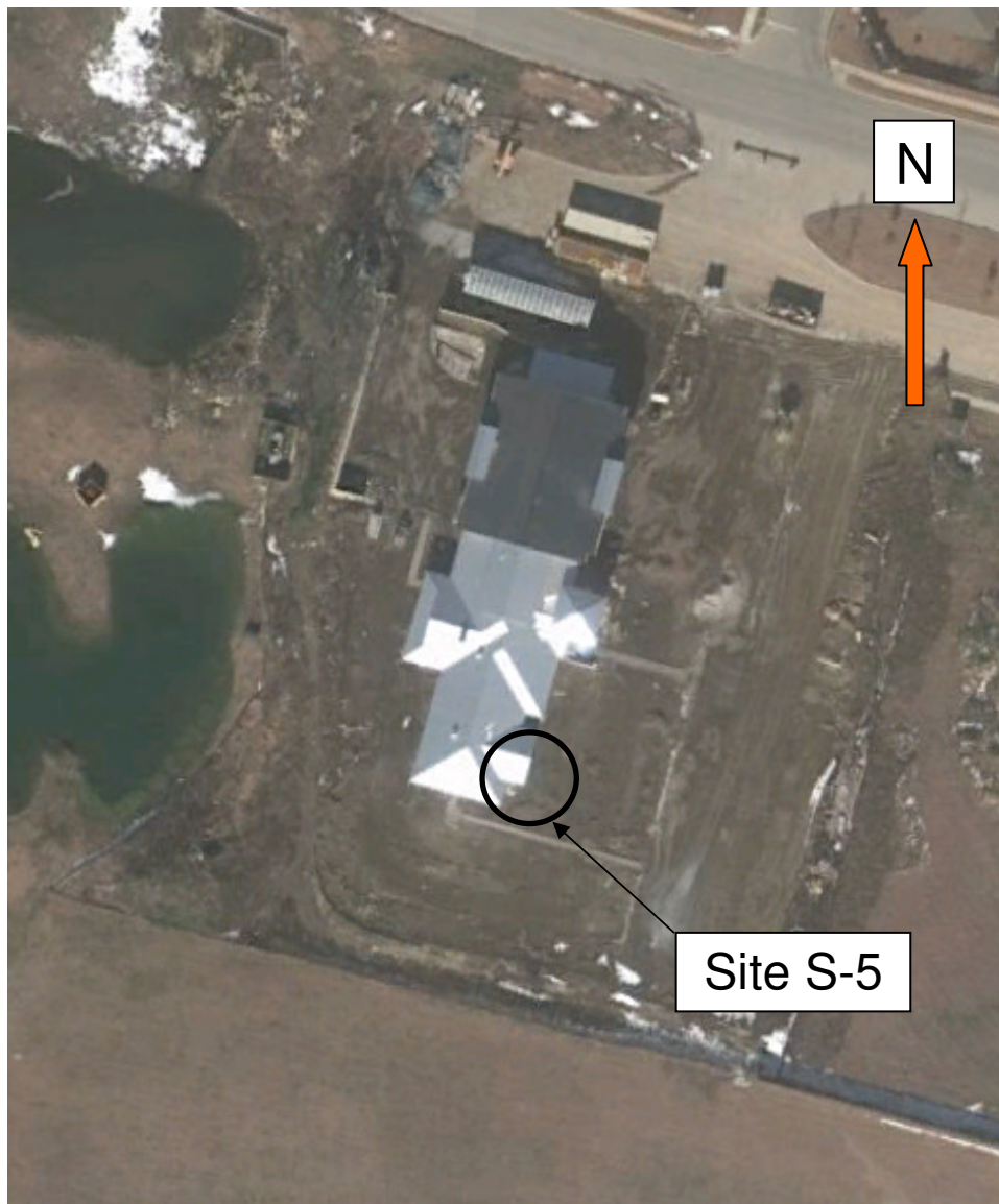
Figure 2.1-8. Aerial Map of Site S-5—Fire Station 34
