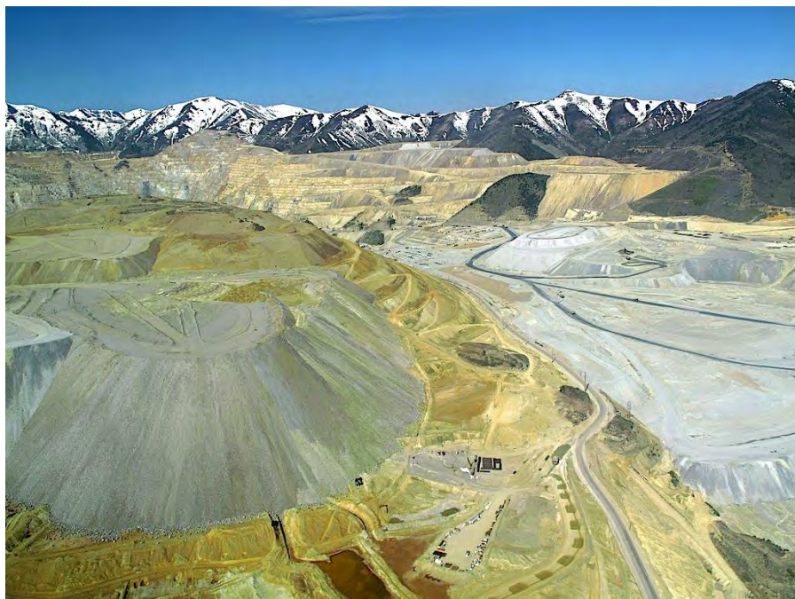
Waste rock dumps surrounding the Bingham Canyon Mine, Utah. Photo by Earthworks.
