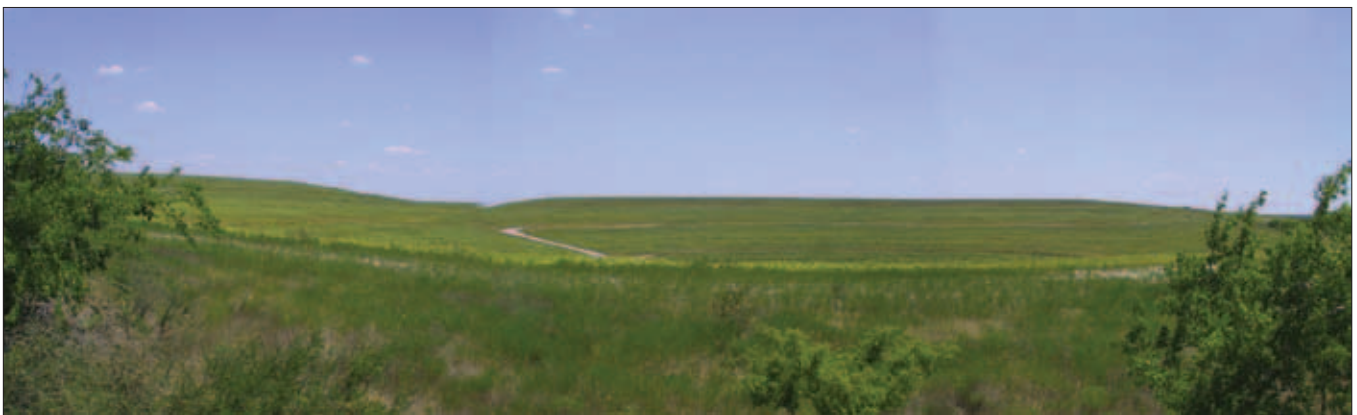
Figure 7-2 Reclaimed Abandoned Uranium Mine—Live Oak County
