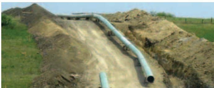
Figure 4-4 Transmission pipeline construction project near Fort Worth
