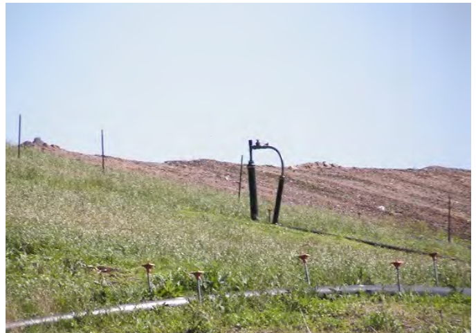
Gas to energy - Denton Landfill
