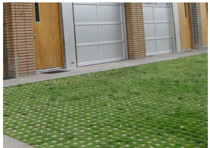
Low-Impact Development - Permeable Pavement
