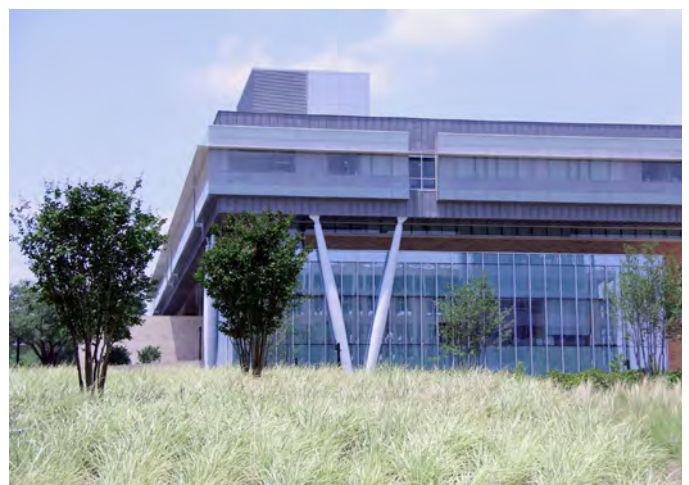
Sustainable Building Design- UNT
