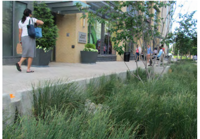
Low-Impact Development - Bioswale
