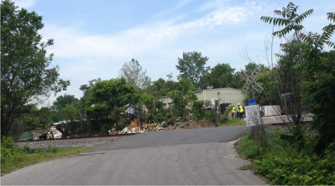
Figure 7. Truck driver's approach view of grade crossing when heading northwestward on private road from carrier terminal (STOP sign not visible).
