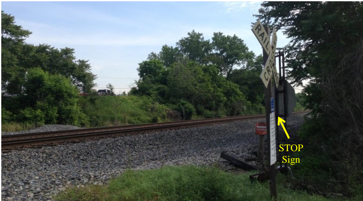
Figure 8. View of STOP sign facing away from roadway, relative to road, railroad, and crossbuck sign.
