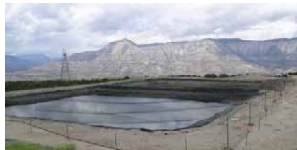
Examples of tanks and pits
