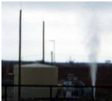
Venting, as shown in this photograph, releases methane and other hydrocarbons.
