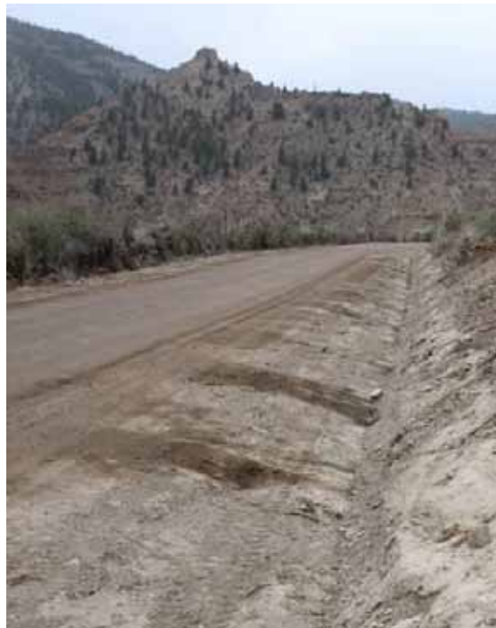
Road with dust suppressant
