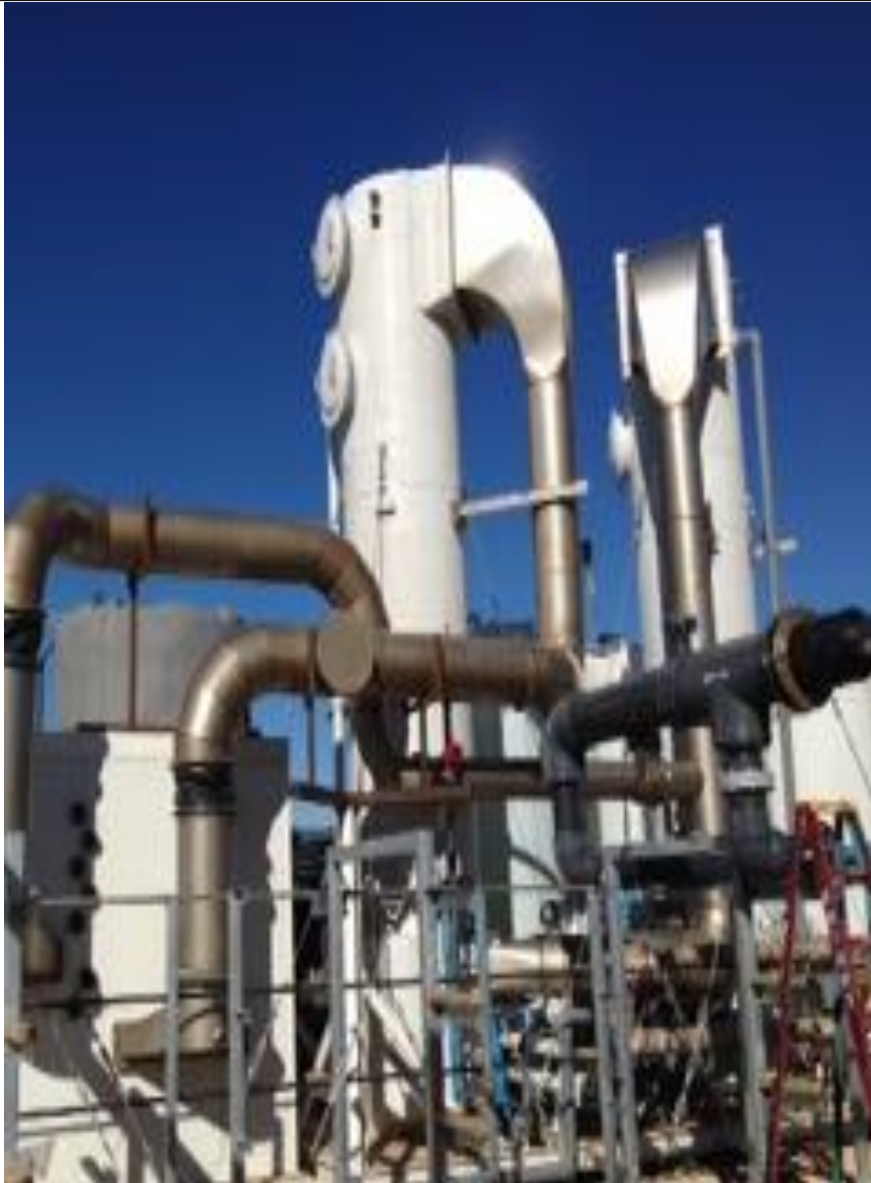
CGE™ Tower at Hutt
