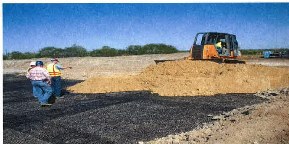
State-Managed Cleanup, Installing a Protective Cap with a Geogrid Support Matrix, Kleberg County, Texas
